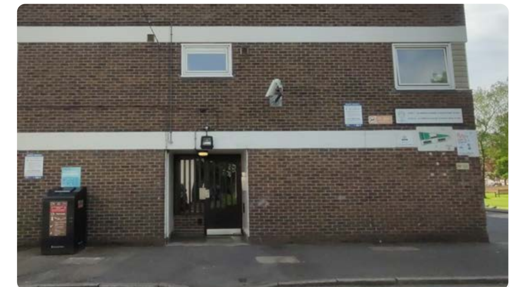
Existing entrance to Lambfold House
