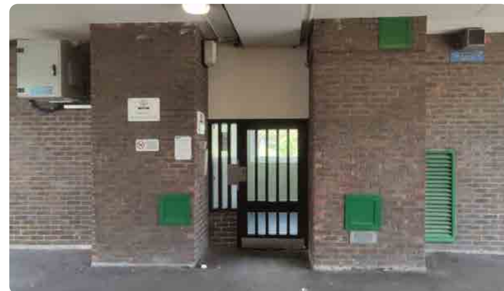
Existing entrance to Kinefold House
