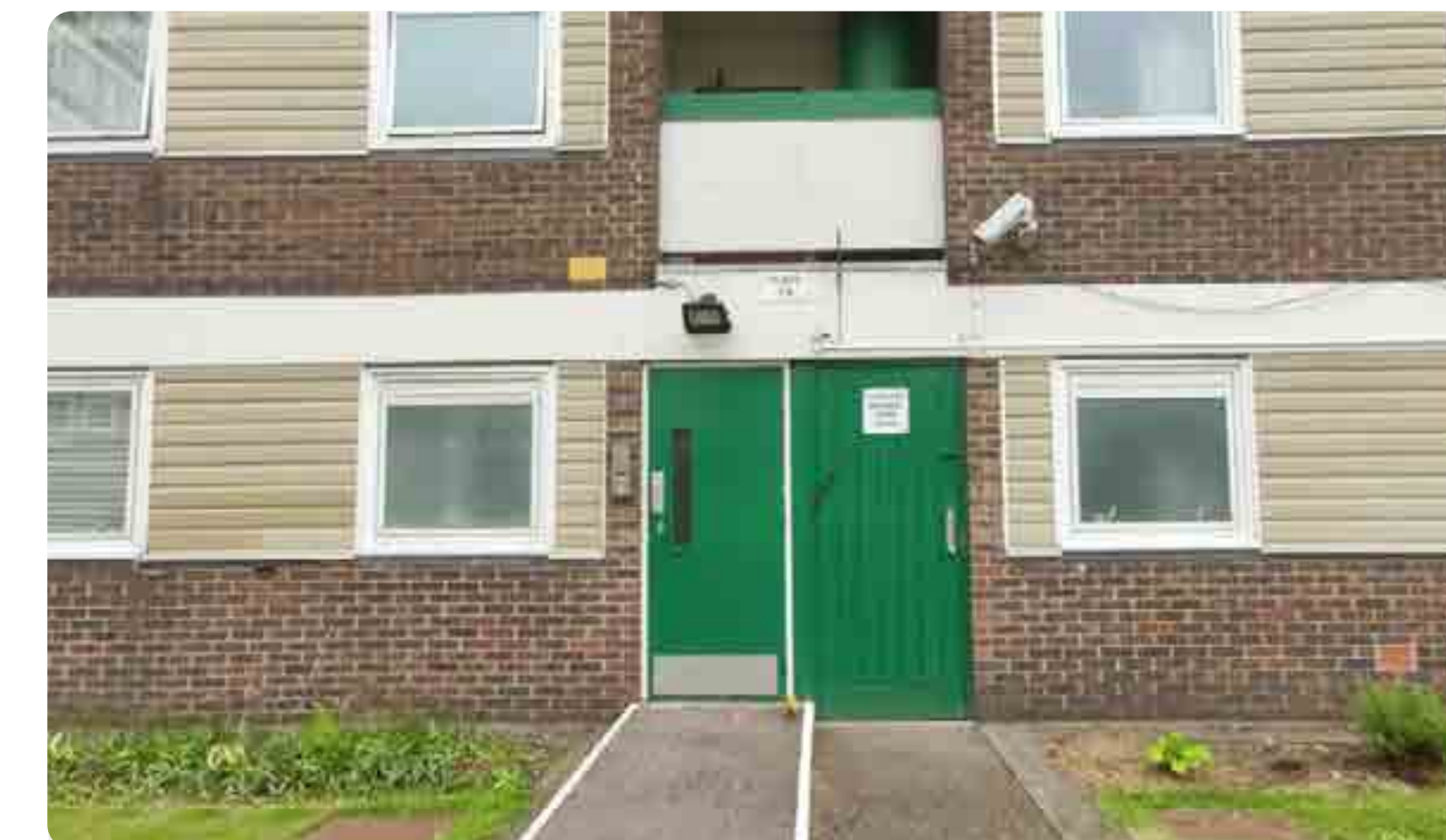
Existing entrance to Shepherd House
